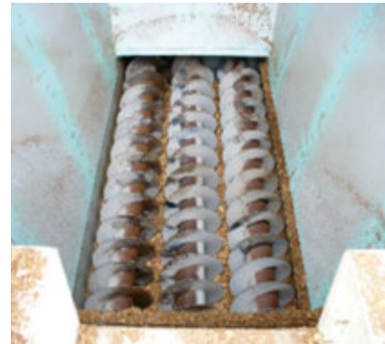
Mounting in discharge screw (wood-fired power plant)
