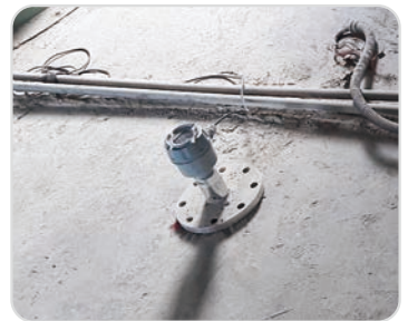
Feeding plant Corn storage tank detection
